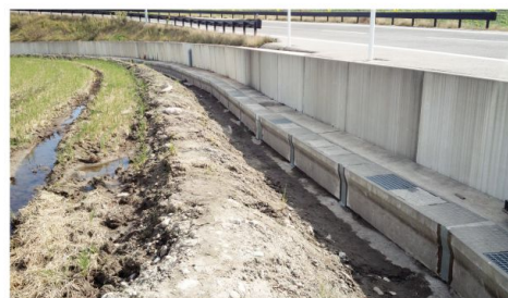
V S側溝目地補修
